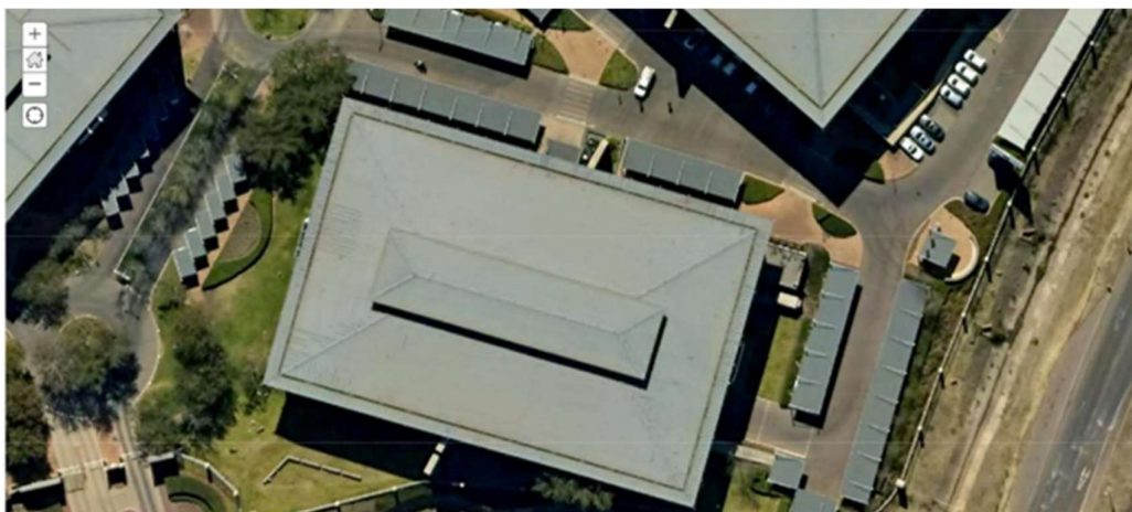
Figure 1 – Aerial View of NNR Building Roof
