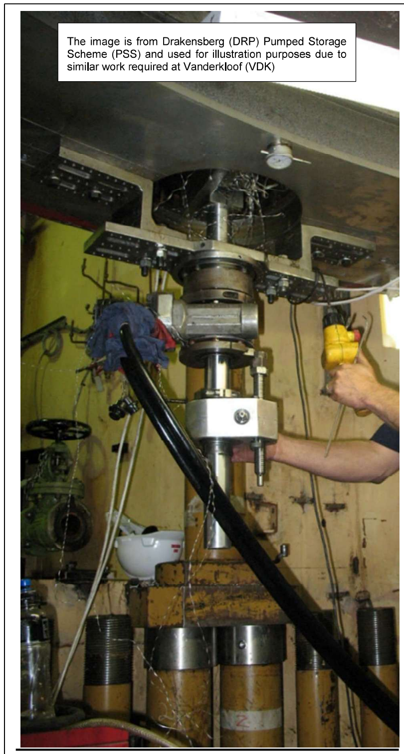
Figure 7: Example of similar guide vane middle bush casing repairs
