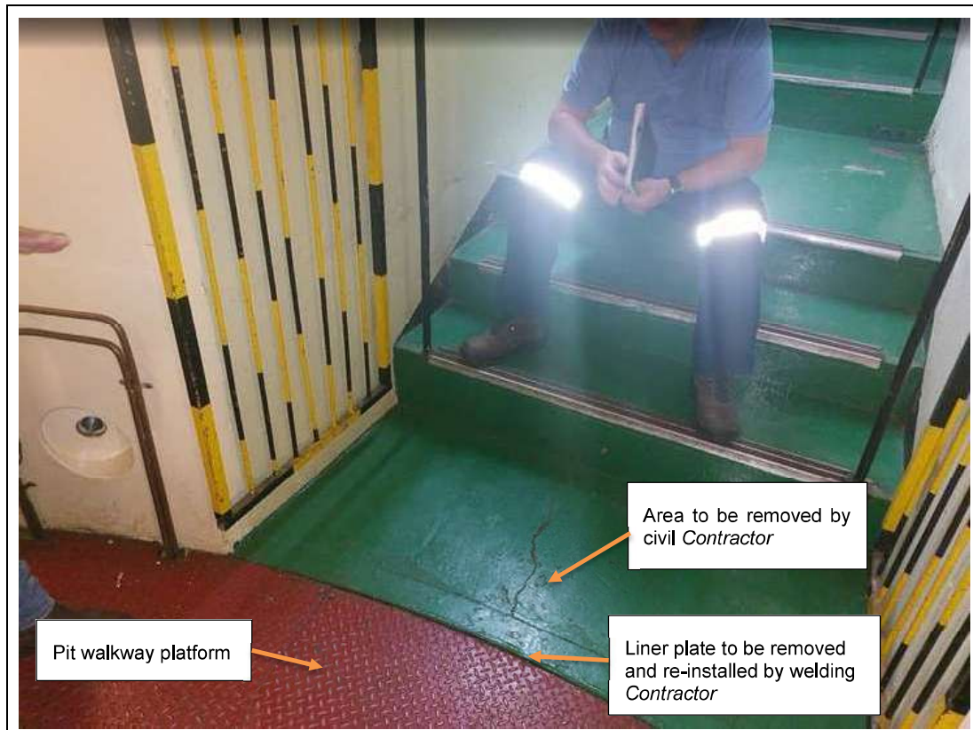
Figure 38: Turbine pit stairway steel liner plate for removal
