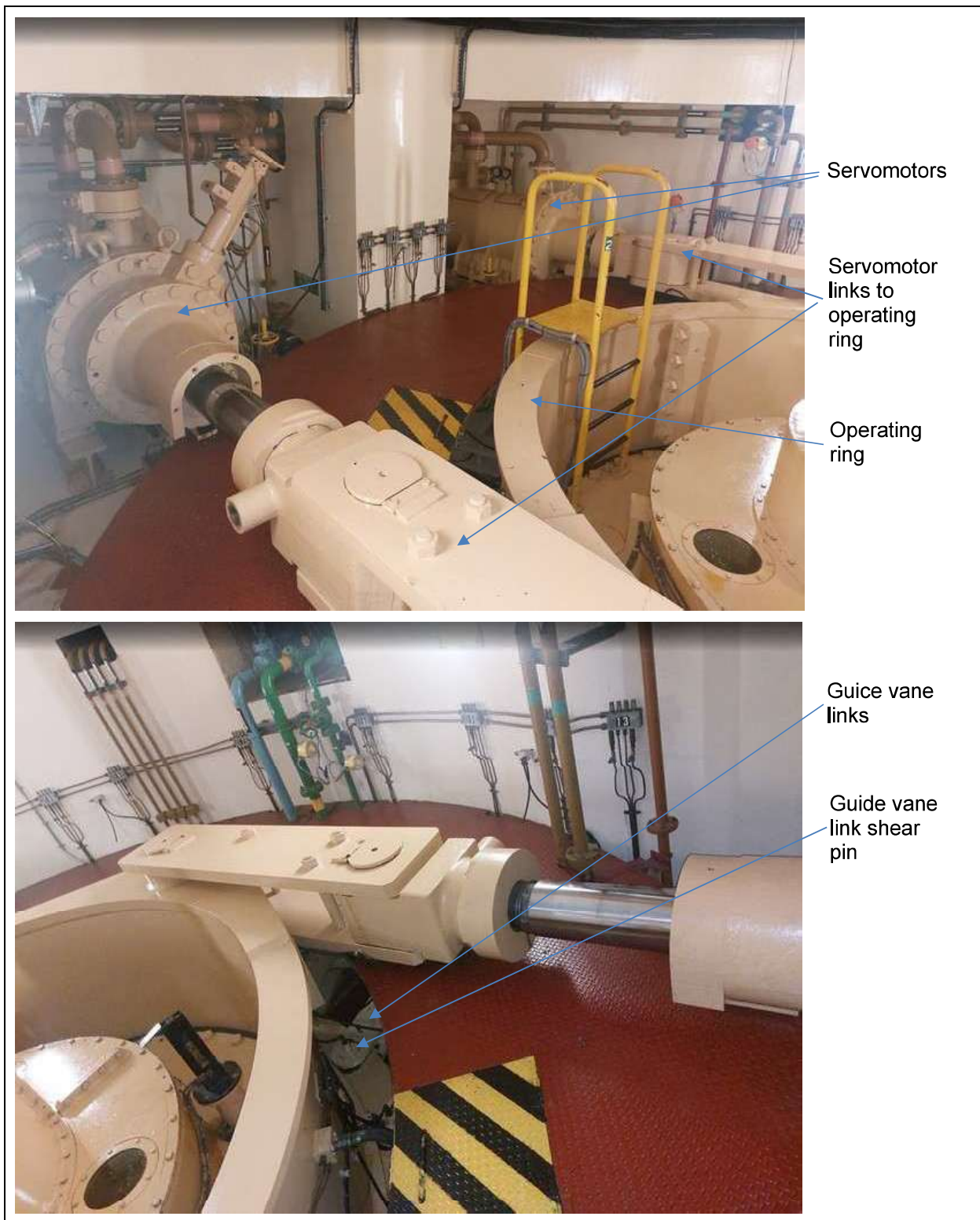
Figure 22: Operating ring and servomotor and guide vane link interfaces
