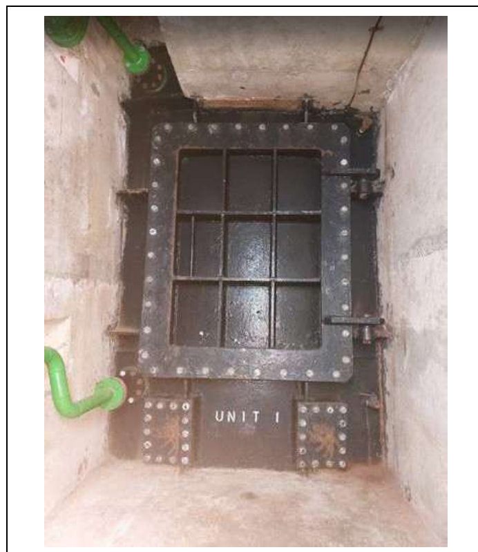
Figure 13: Draft tube access mandoor in closed/seal condition with draft tube charged
