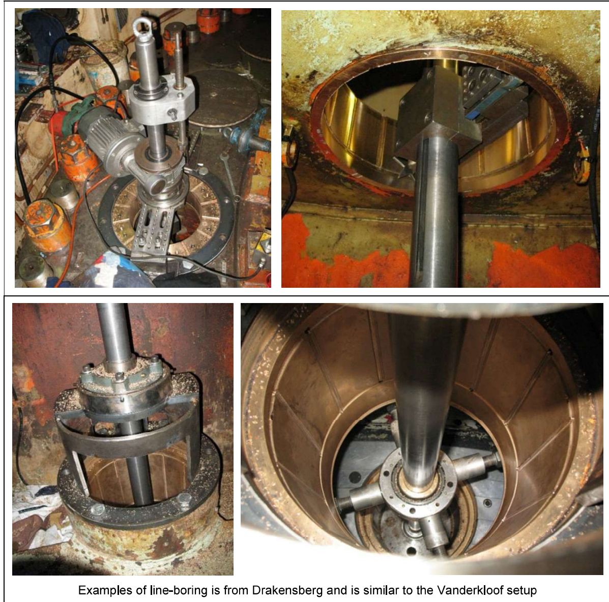
Figure 45: Examples of line-boring setups for the bush casing internal machining
