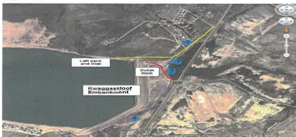
Figure 3: Plan view of Kwaggaskloof embankment (Google Earth, 2013)
