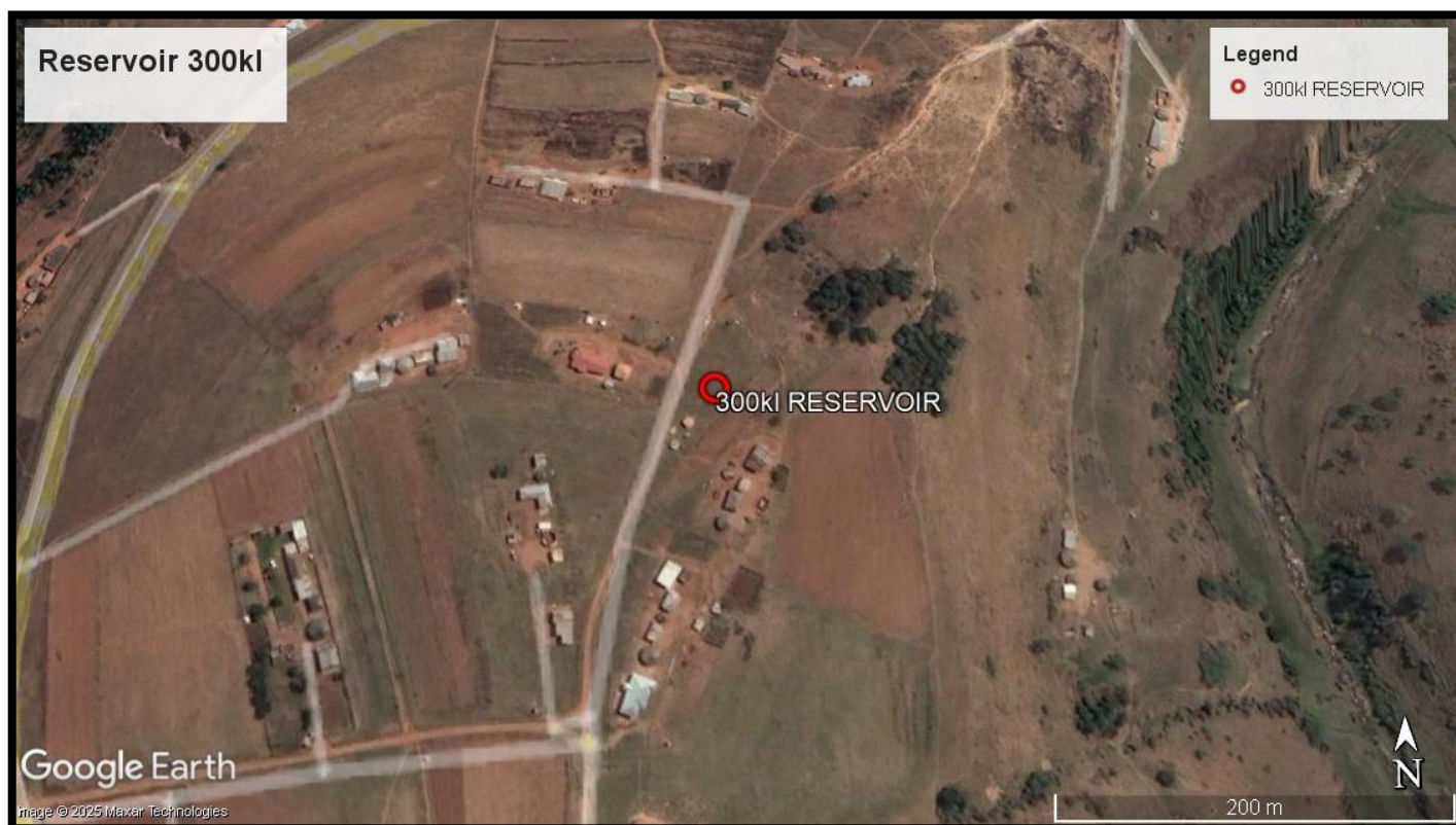
Figure 2: Location of 300kl Reservoir- 29° 4'22.60"S , 29°30'47.38"E
